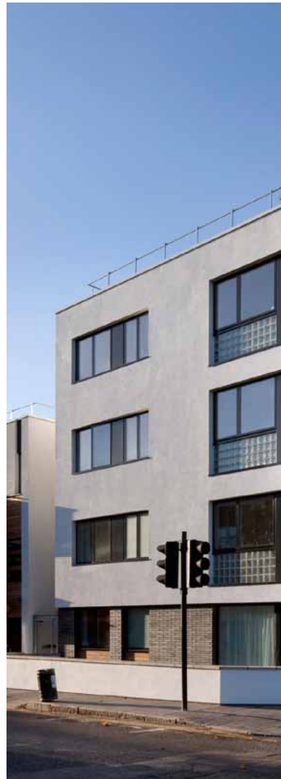
Below: Boleyn Road apartments
