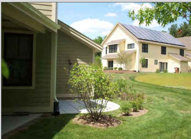
Note composition of buildings on the land that are arranged with the topography and angled orientation to create private and common spaces
