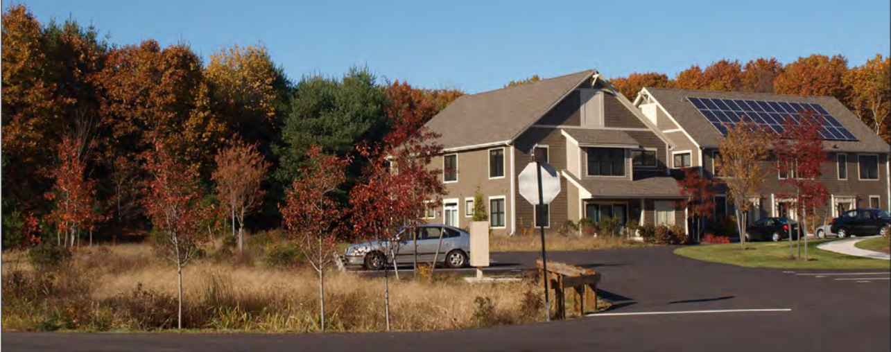
Vegetated drainage basin provides a different buffer
