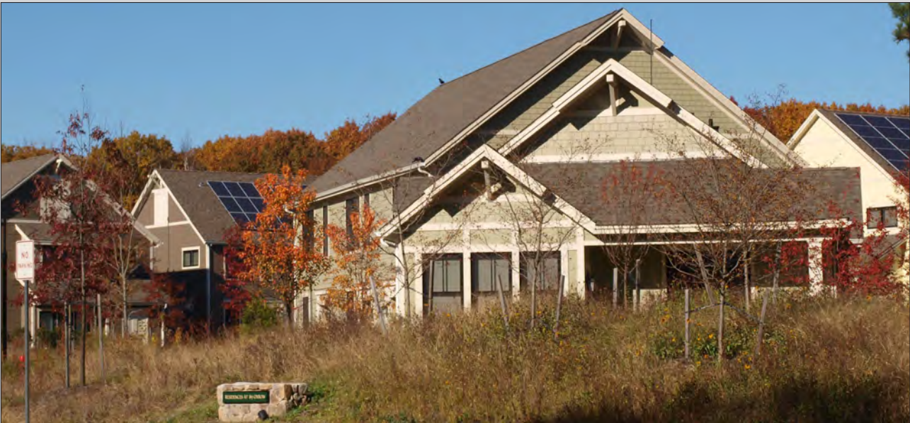
Vegetated mound along frontage softens visual impact of building
