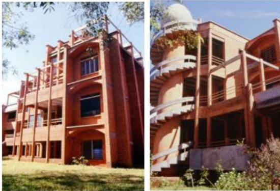
13 apartments on 4 floors 'ater tank tower with staircase
