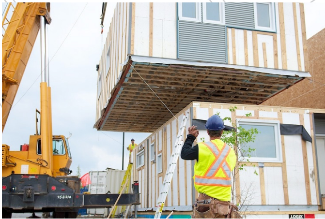
Figure 3.9 Custom-Built Modular Homes by SMLy Mod Prefab Homes, Canada
