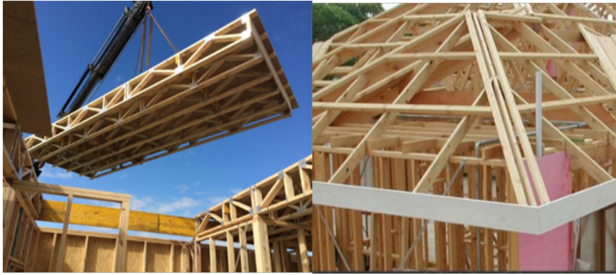
Figure 2.7 Timber Framing System
