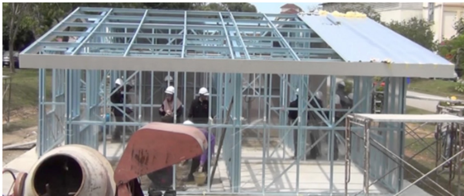
Figure 2.6 Metal Framing System
