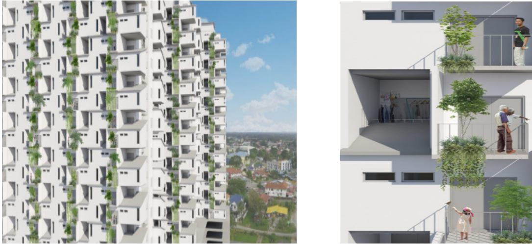
Figure 2.35 Greenery Façade and Built-in Planter Box at Balcony
