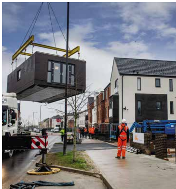
Ilke Homes module installation
