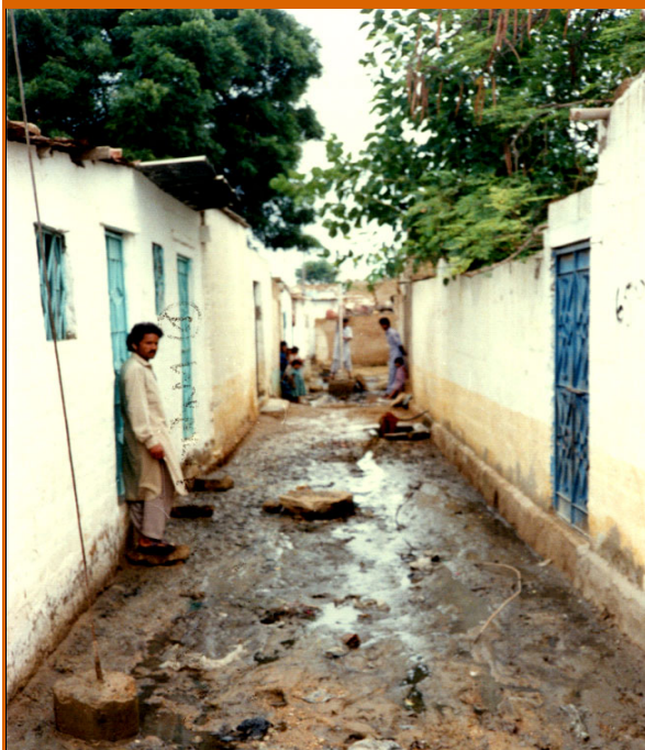
The sewage problem
