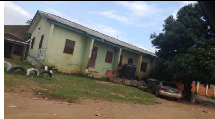
Plate 2: The FHA lugbe is in a poor state of infrastructure. The scheme is mostly without access roads, and not connected to the central sewage system
