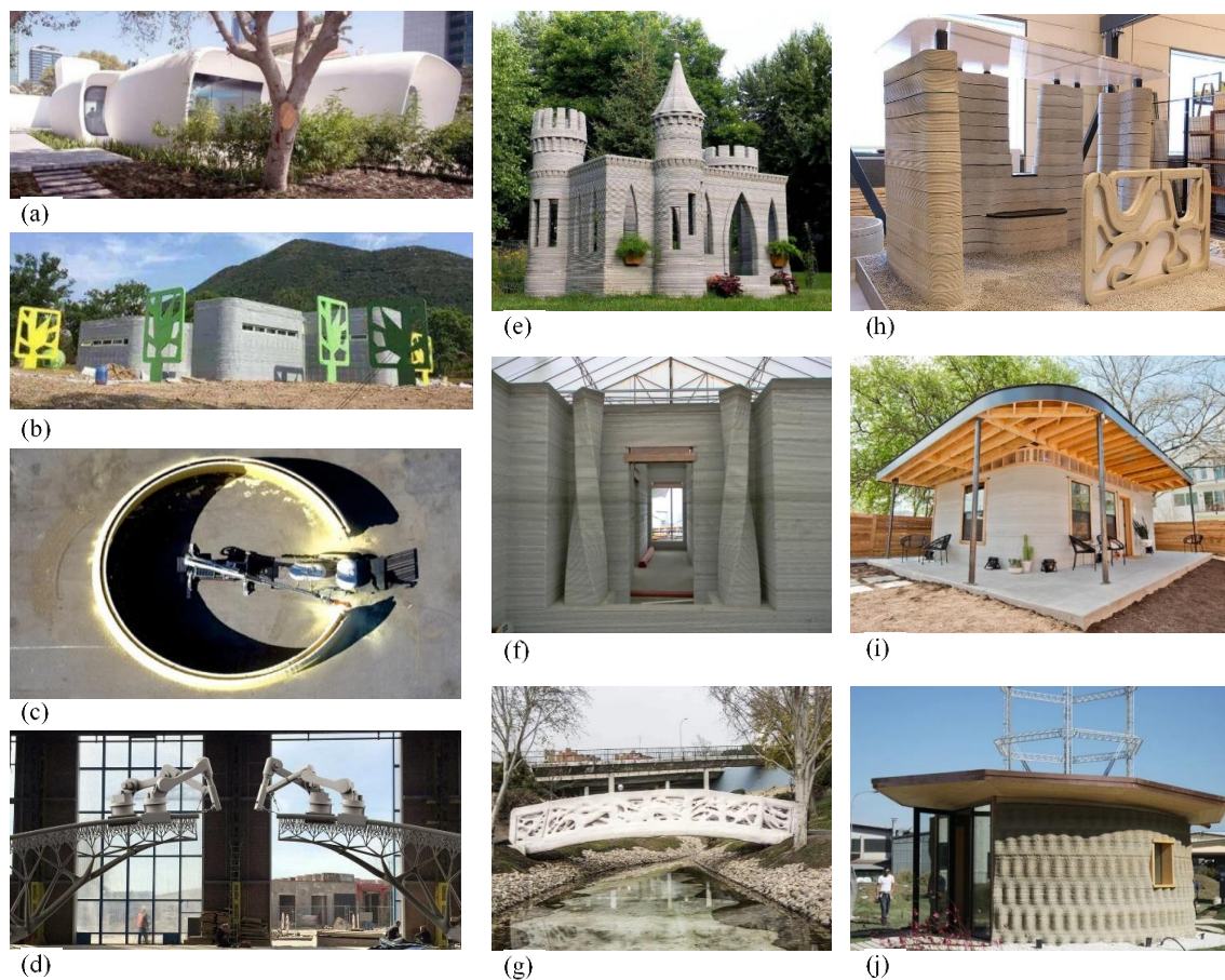
Figure 3. 3D-printed construction projects around the world (derived from [71–80]): (a) Office building in Dubai, UAE, completed in 2016; (b) Public restroom in Da Yang Mountain, China, completed in 2016; (c) 12-foot dome in California, USA, completed in 2017; (d) MX3D bridge in Amsterdam, Netherlands, completed in 2018; (e) First 3D-printed Castle in Minnesota, USA, completed in 2014; (f) Hotel in Manila, Philippines, completed in 2015; (g) Pedestrian Bridge in Madrid, Spain, completed in 2017; (h) TU Eindhoven Pavilion, Netherlands, completed in 2016; (i) Home for vulnerable people in Tabasco, Mexico; and (j) 3D-printed house with natural soil in Italy, completed in 2018.
