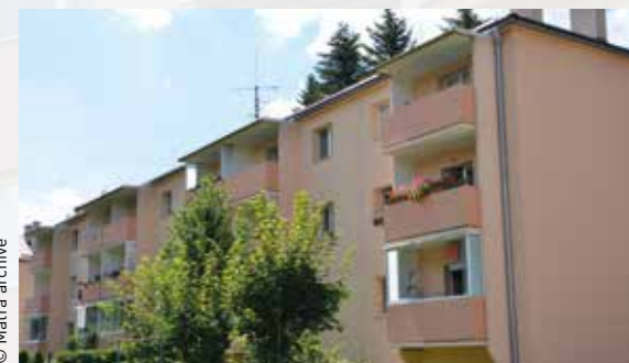
Renovated and modernised building
