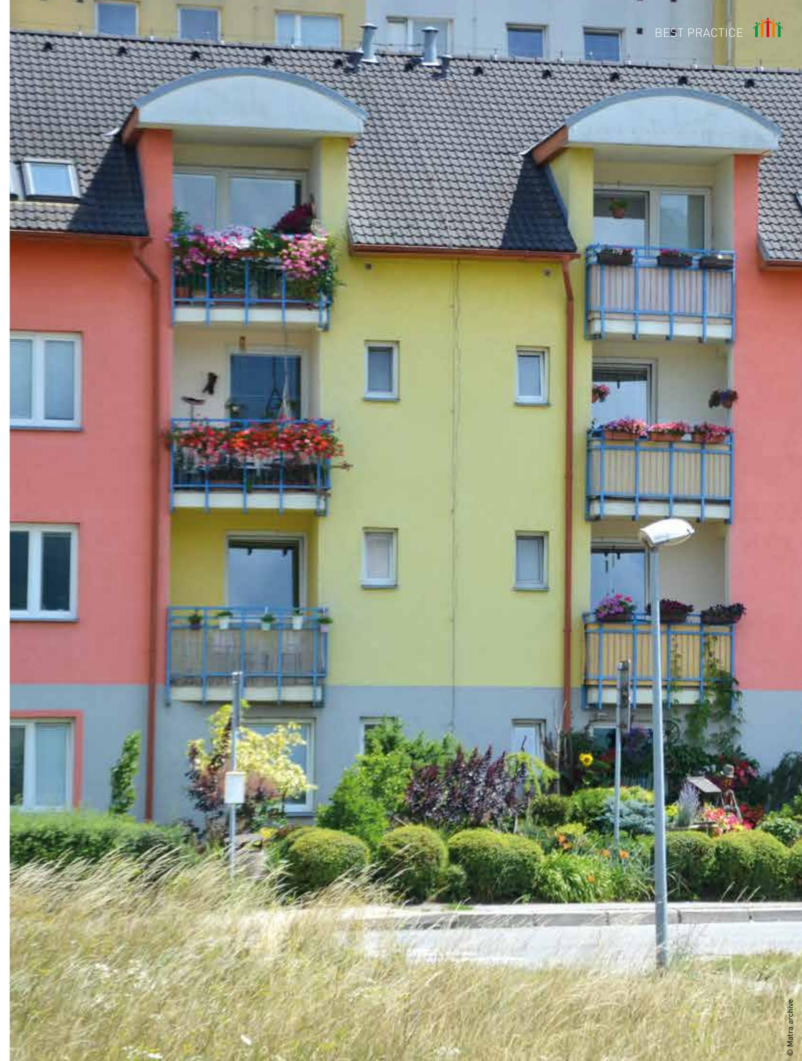
Renovated and modernised building
