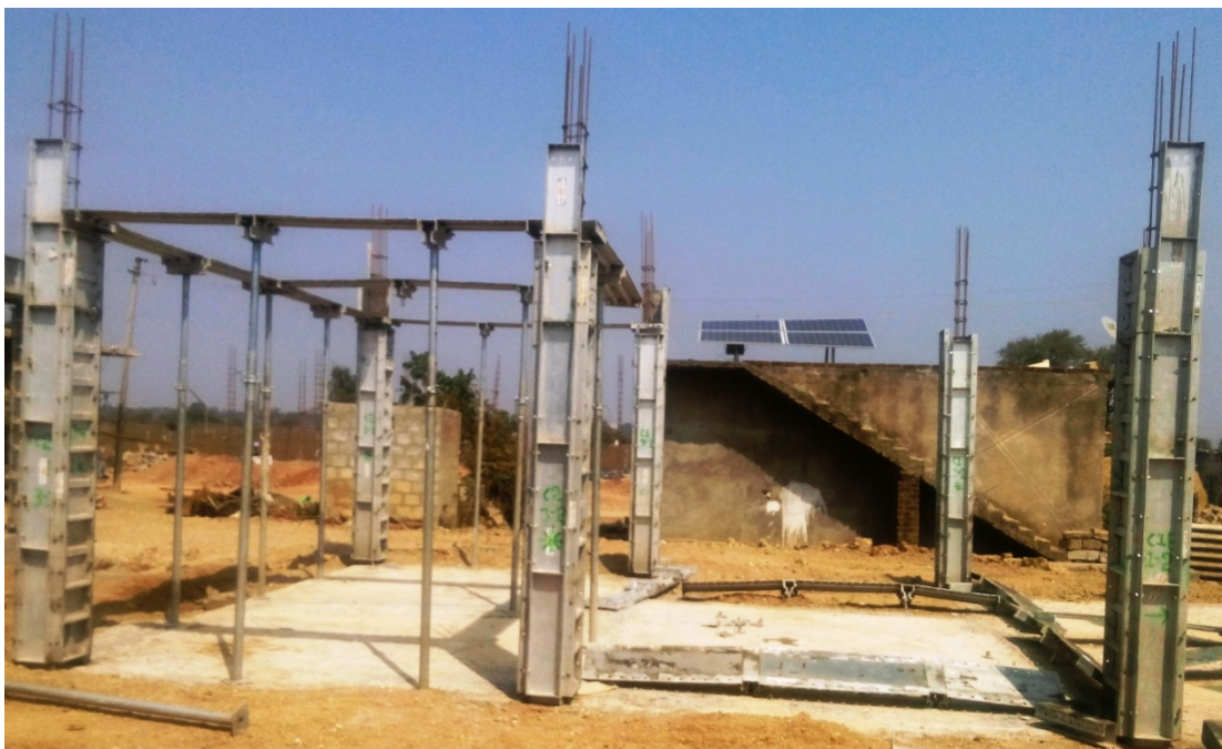
Figure 3. Special aluminum form work used for casting concrete.
