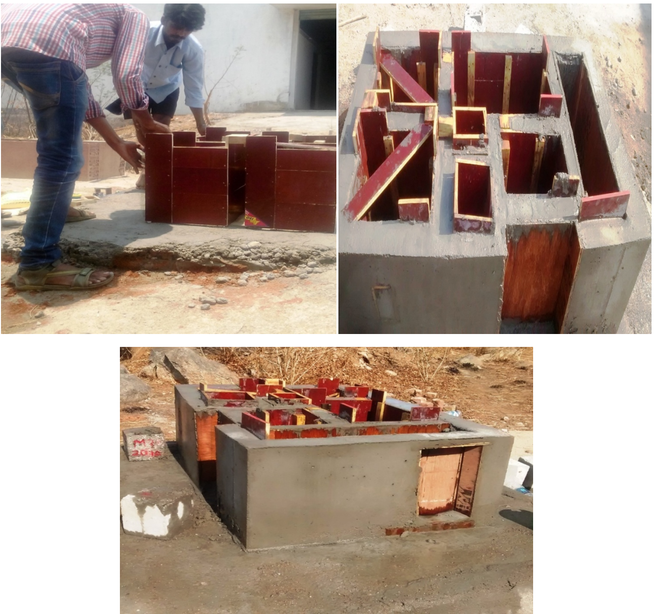
Figure 1. Proto type of the modal house filling with concrete.
