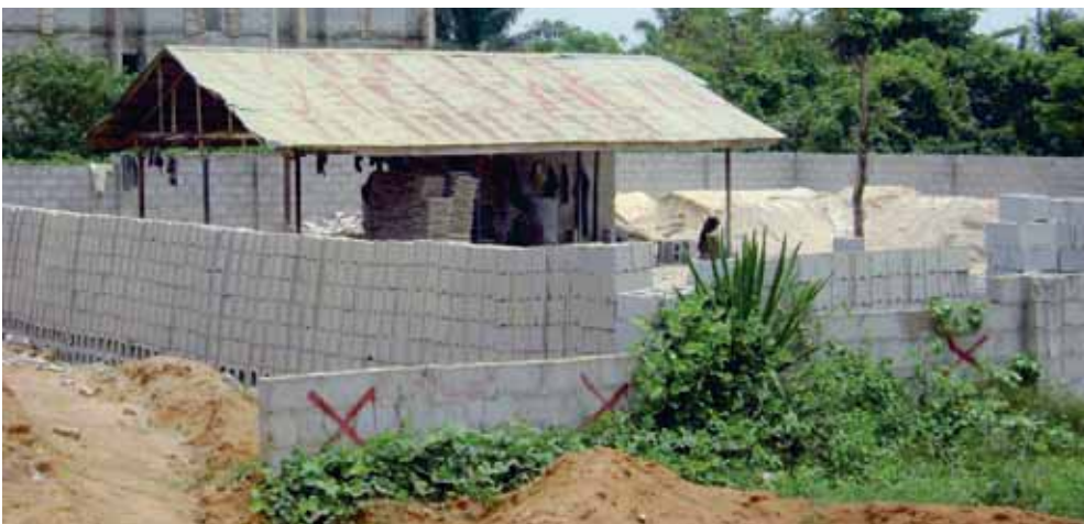
Figure 27: Block construction, Nigeria. Photo © UN-HABITAT/ Claudio Acioly
