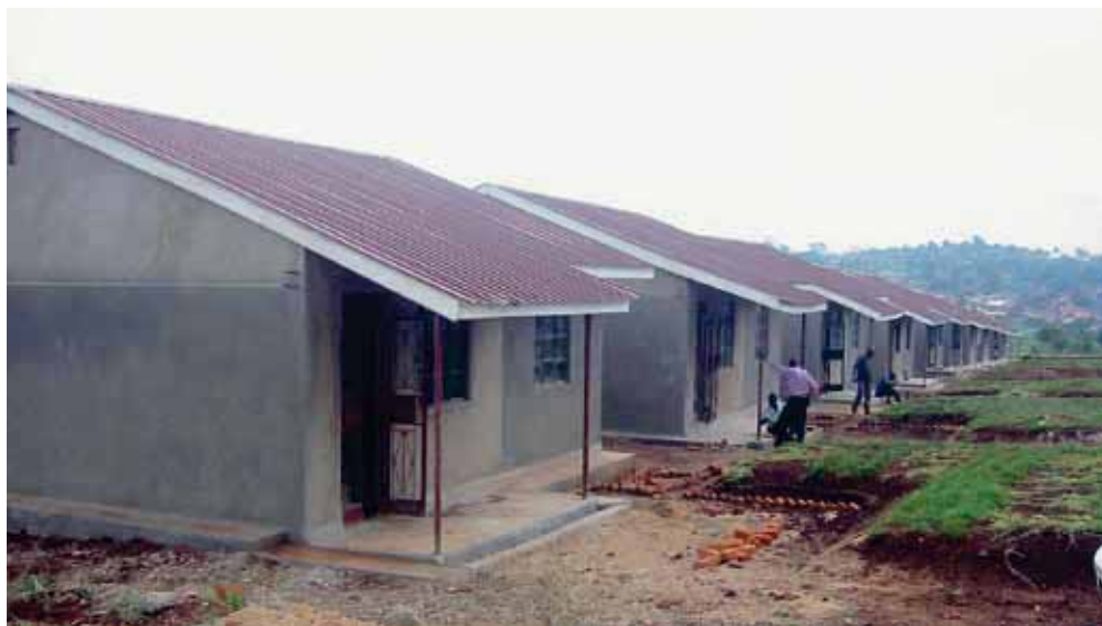
Figure 24: Self-help houses nearing completion in Uganda. Photo © Suzi Mutter
