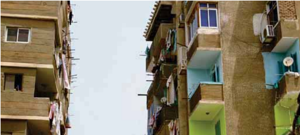
Figure 13: Six-storey apartment buildings in Egypt. Photo © UN-HABITAT/Matthew French
