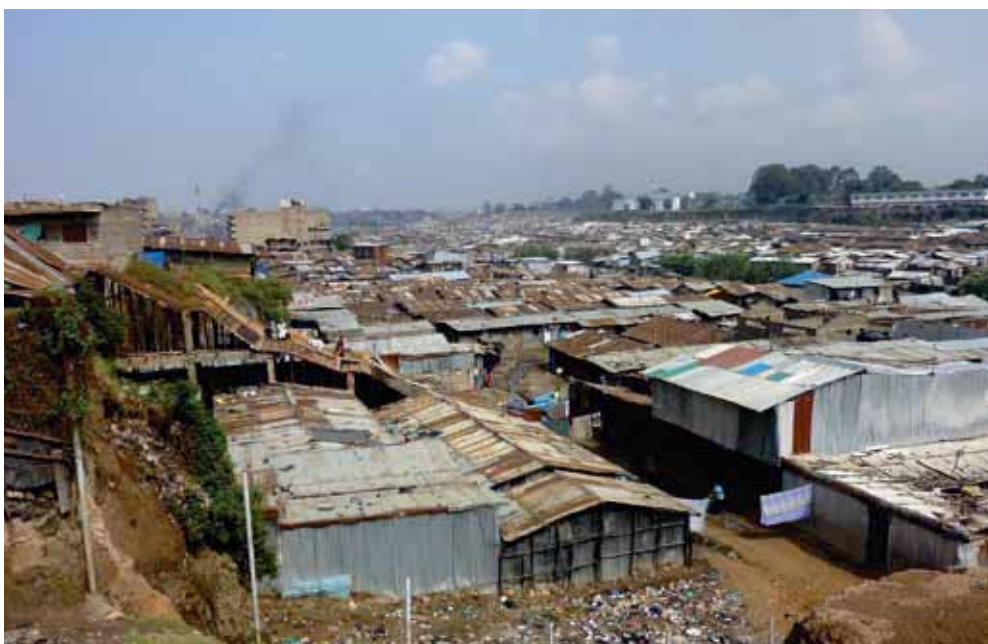
Figure 15: The informal housing landscape in Mathare Valley, Nairobi, where much of the housing stock is rental housing. Photo © UN-HABITAT/Matthew French
