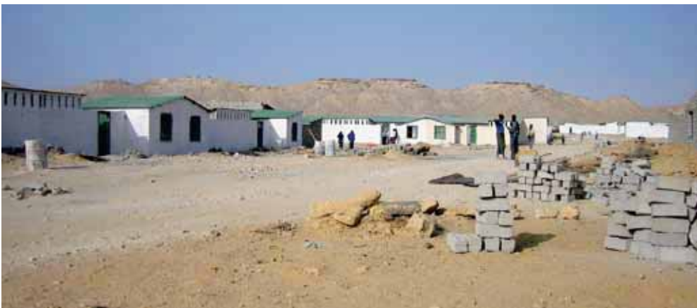
Figure 31: Housing development in Somalia. Photo © UN-HABITAT
