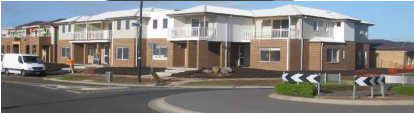
60 units in Brimbank Gardens, Victoria
