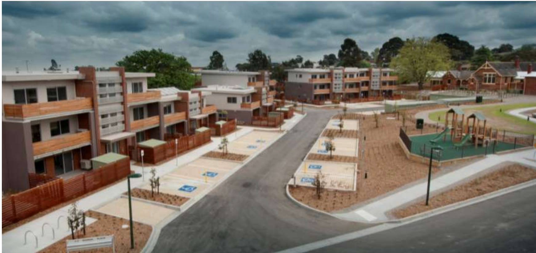
CHL's 79 units Affordable Housing Development
