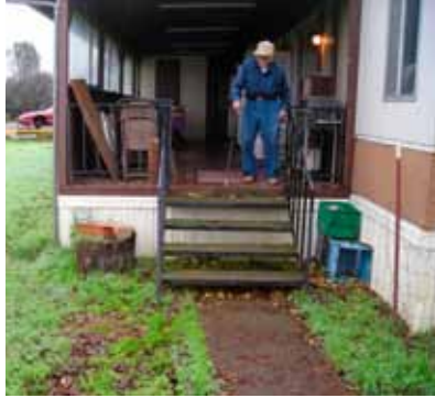
A steep staircase poses a danger to this elderly resident.
