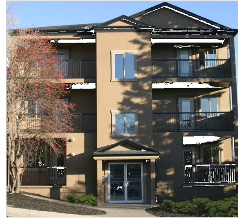
Above: Image 27 - Alberta's first Energuide rated building with an Energuide rating of 88 & it meets R-2000 criteria. Using insulated concrete forms (ICF) and triple pane windows to produce a superior building envelope. It has solar power, energy start rated appliances, water saving fixtures/toilets and a low maintenance exterior.
