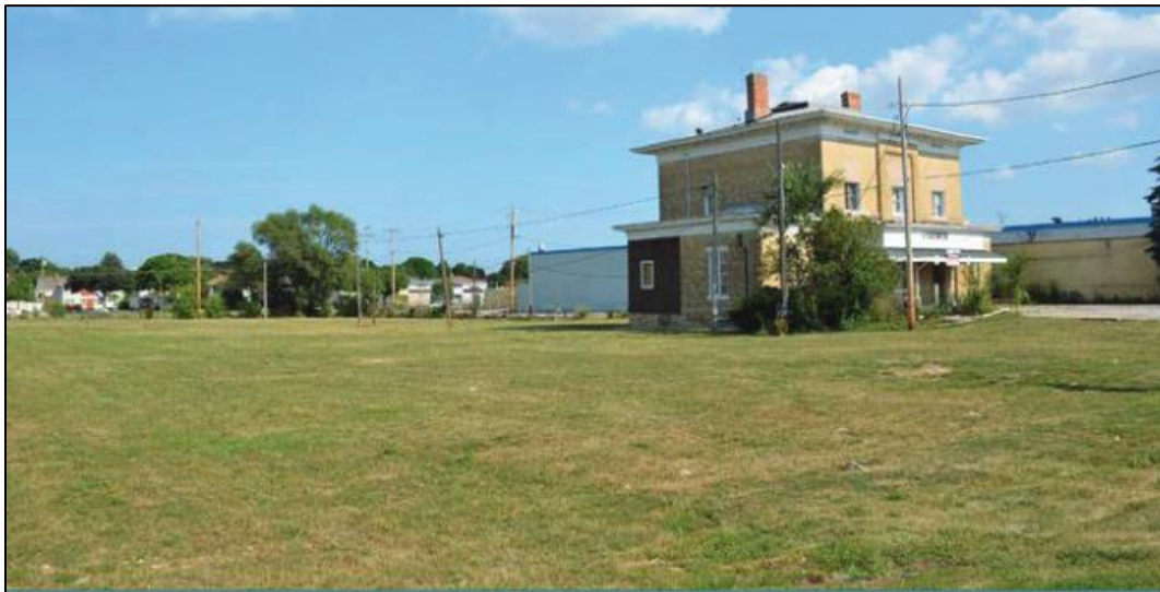
Figure 8: Former Wildenberg Hotel at 3447 S. 27 th Street Source: City of Milwaukee
