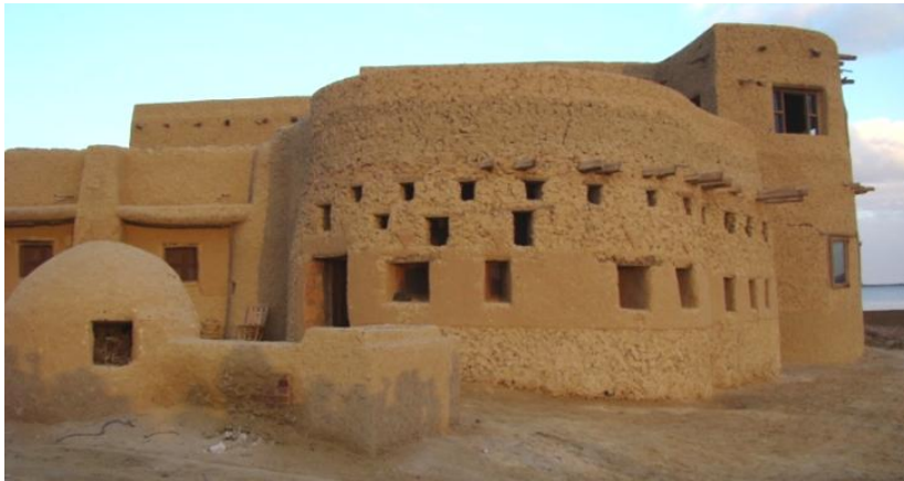
Figure 27: Adrere Amellal eco-lodge in Siwa Oasis built using traditional Siwan building materials and techniques. Project architects: EQI 21
