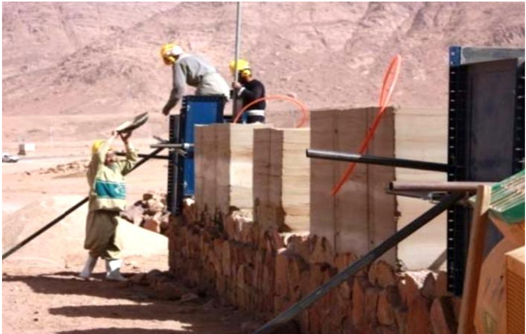
Figure 41: Rammed earth construction in Saint Katherine. 33
