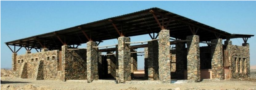
Figure 25: Visitors Center in Wadi Al-Gemal protectorate in Marsa Alam constructed with local stone bearing walls and corrugated sheet roofs. Project architects: EECA 19 .
