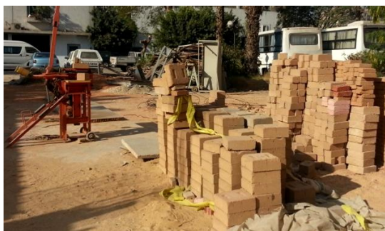
Figure 34: CSEB blocks produced at the HBRC headquarters.
