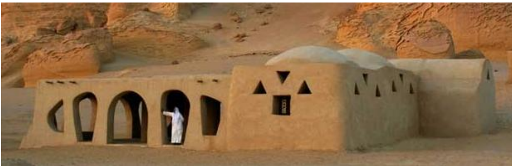
Figure 26: Visitors facilities at Wadi AL-Hitan protectorate in Fayoum constructed with adobe bricks bearing walls, domes and vaults from local desert clay. Project architects: Eco-Architecture 20
