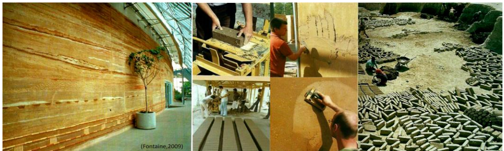
Figure 8: Different techniques of earth construction: CEB, Rammed earth, Adobe and wall plastering. (Fontaine, 2009)
