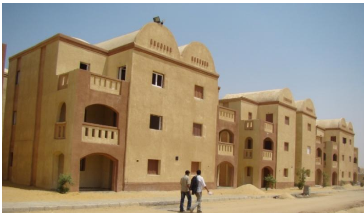
Figure 50: Residential buildings with vaulted roofs in Haram City.
