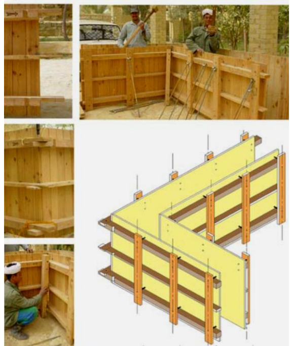
Figure 33: Wooden shuttering for rammed earth. Image courtesy of architect Adel Fahmy.
