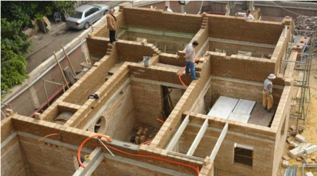
Figure 36: Construction of experimental building at the HBRC (Farouh, 2012).
