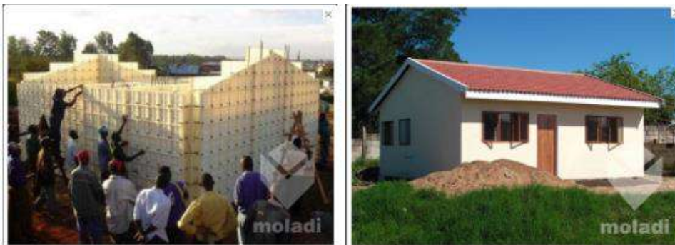
Figure 4: Construction with Moladi Plastic Panels (Moladi, 2018)
