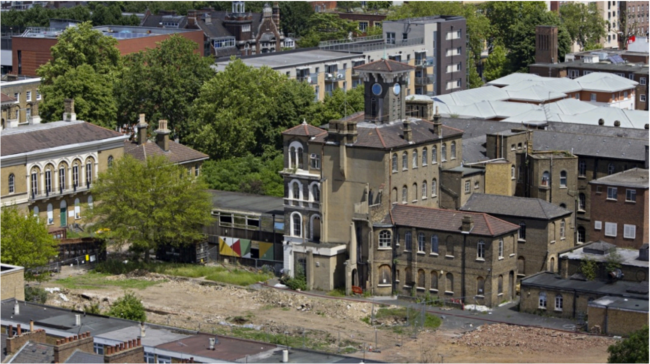
Figure 4.3.1: A photograph of the former St Clement's hospital in Mile End, the site of London's first CLT. Source: http://www.theguardian.com
