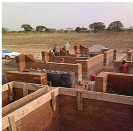
Fig 2:- House under construction in Zambia
