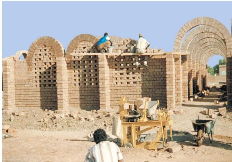
Fig 3:- Construction Site in Sudan Observe the Arches
