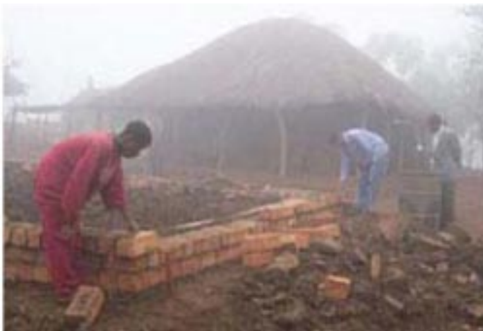
Fig. 3 - A house built of stabilised-soil block and an old style straw-roofed shelter.
