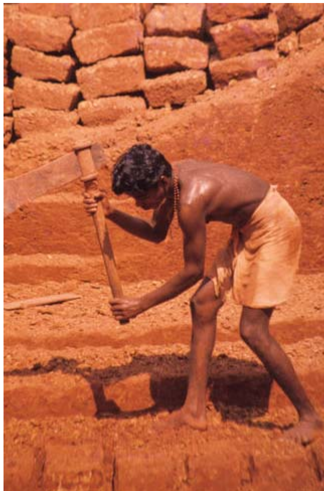
Figure 9 – Quarrying crude laterite building blocks.
