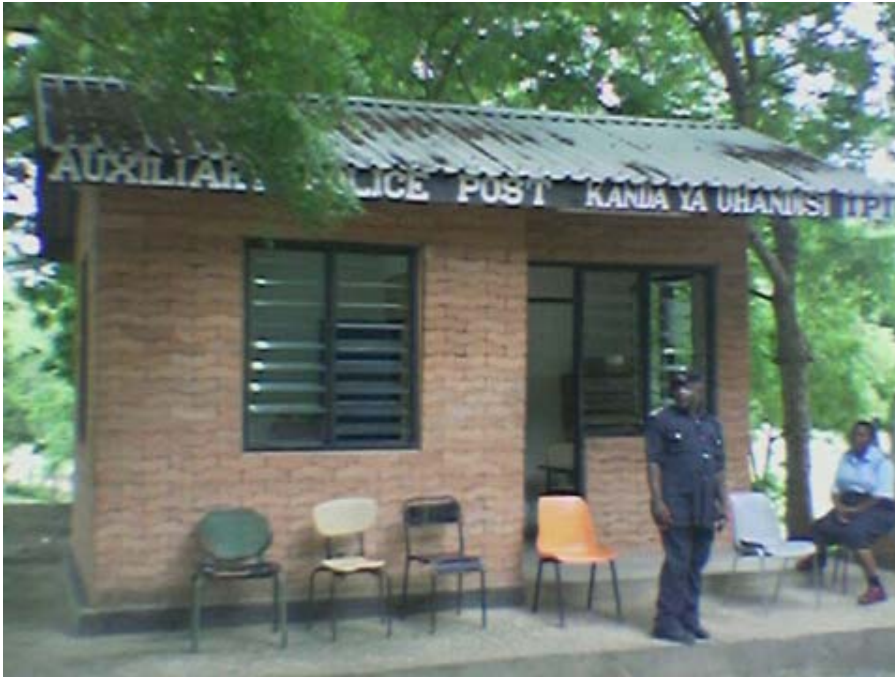
Figure 6 –Guards' house, made of stabilised earth blocks
