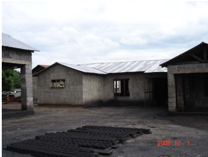
Figure 43. Buildings being completed for a settlement
