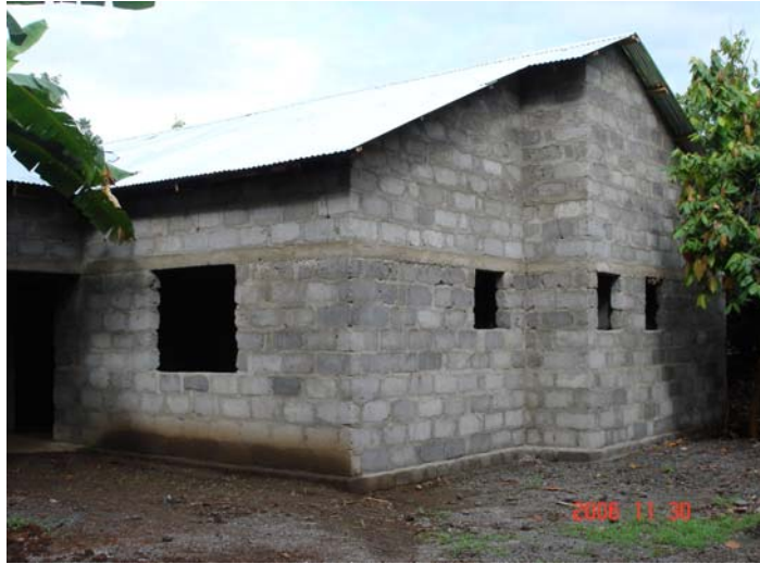
Figure 45. Buildings being completed for a settlement
