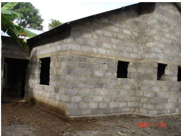
Figure 44. Buildings being completed for a settlement
