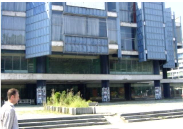
Figure 27. Sarajka mall before demolition
