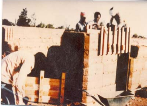
Figure 10. Rammed earth wall construction
