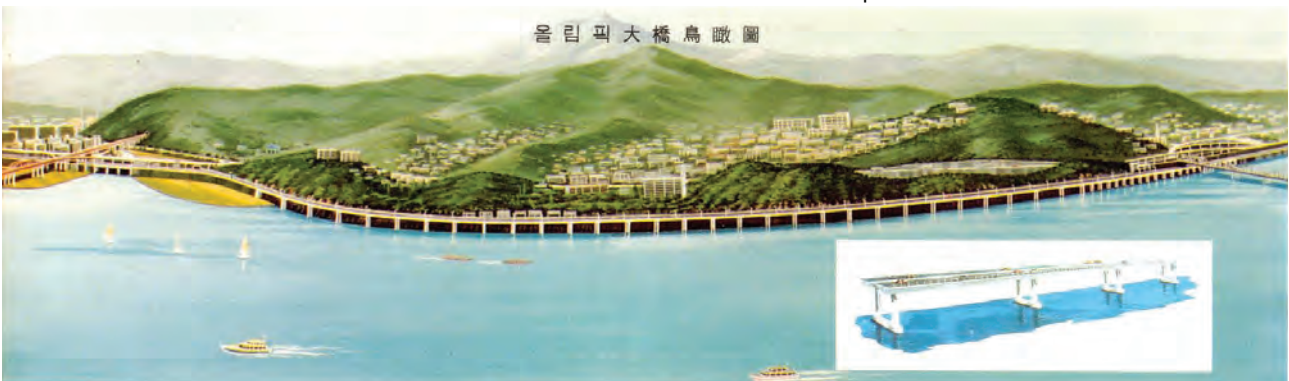
Figure 3-40. Han River Development Project, 1981-86. Elevated portion of the Olympic Expressway along the southern bank of the river. Source: Seoul Metropolitan Government.
