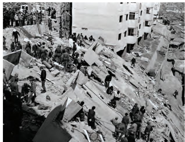
Figure 3-27. Waw apartment collapse rescue efforts, 1970.
