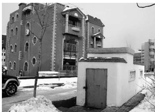
Figure 3.6 Temporary Rubbish Storage Space
