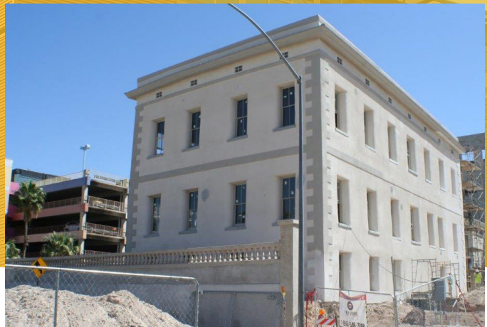
The transformation of Marist College into affordable housing - Tucson, AZ
