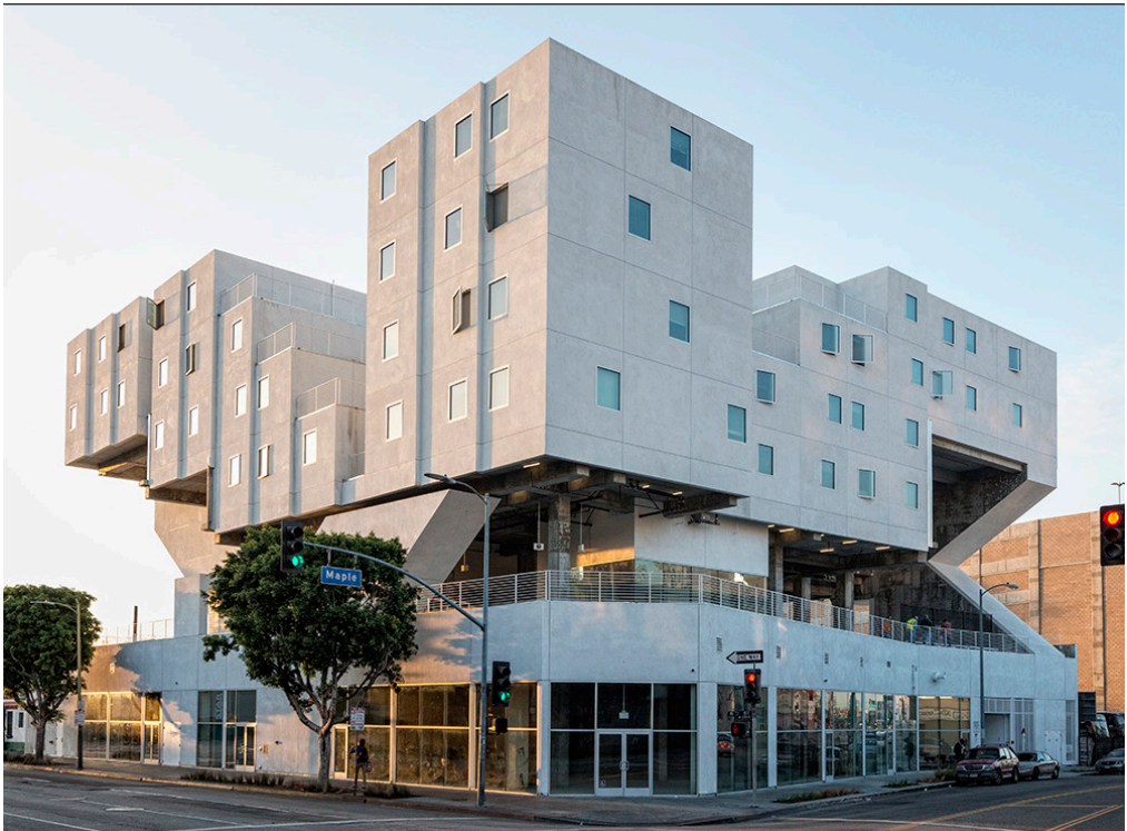
Source: Skid Row Housing Trust
