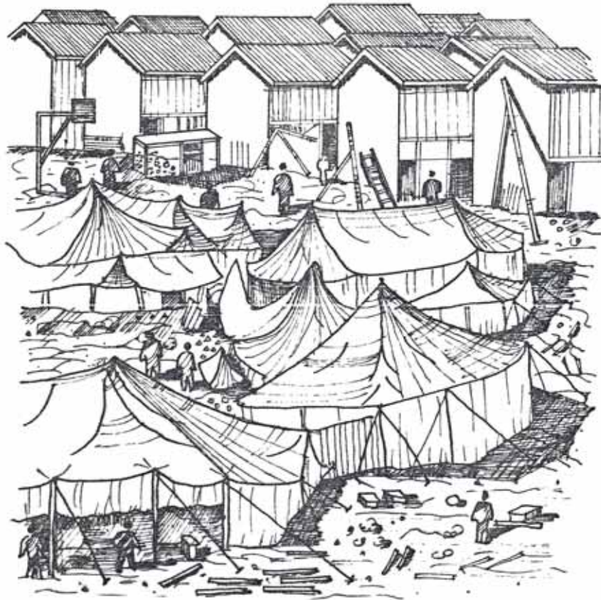
Fig. 2.19 The community lived in tents while they constructed their houses (Ref. 28).
