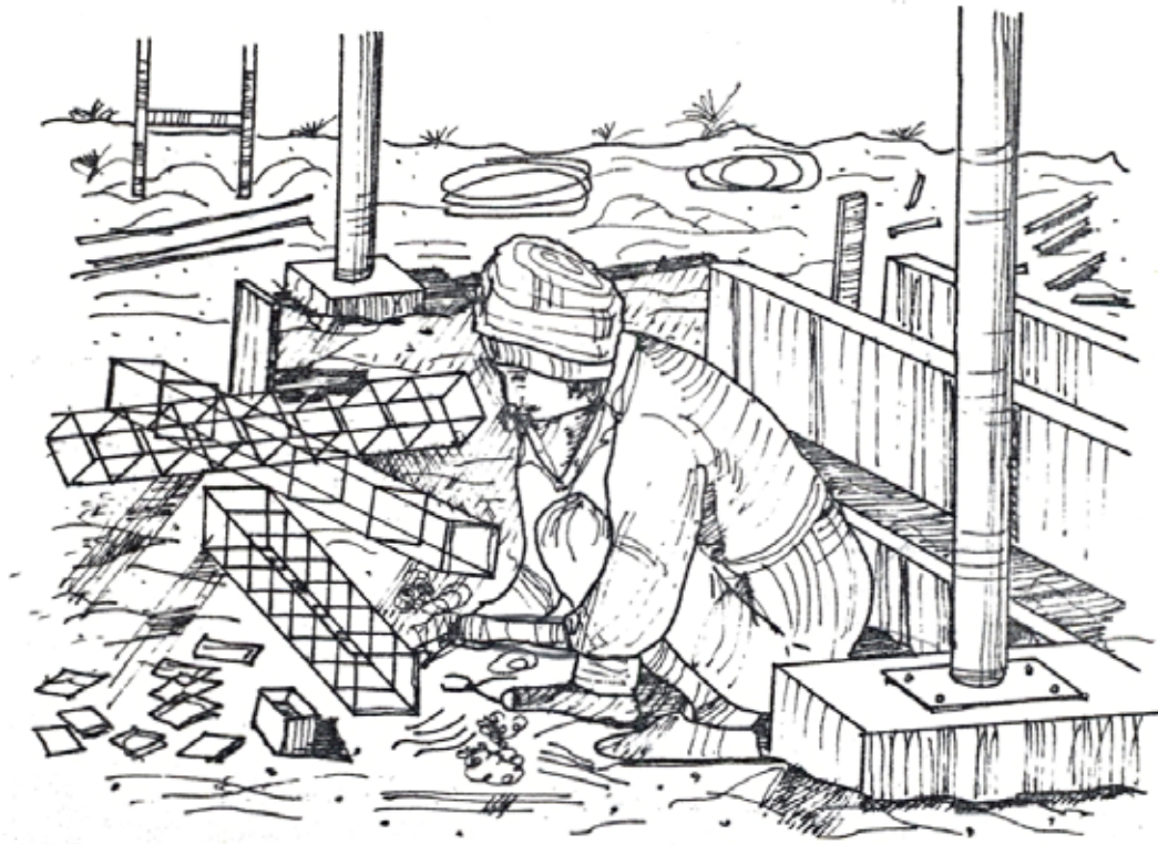
Fig. 2.14 A Participant does rebarring work for pile fabrication (Ref.28) .
