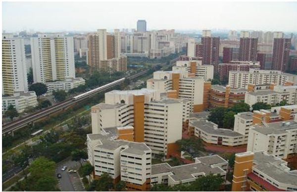
Overview of Bukit Batok, an example of a satellite town developed by the HDB since the 1970s.
