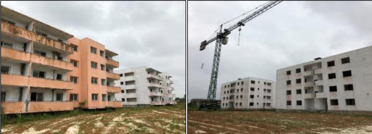
Figure 10. Abandoned construction site and unoccupied buildings at Okala
