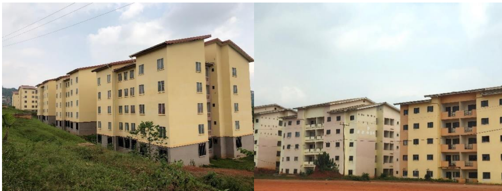
Figure 5. Occupied and unoccupied buildings at the Olembe site
