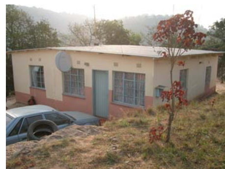
The expected rush for formal financing did not materialise – one of the houses which did not apply
