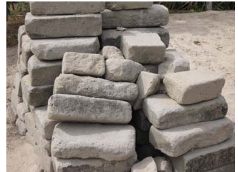
The service offered by CEMEX solves this problem – savings, in the form of concrete blocks, deteriorate due to poor storage
