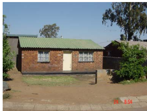
The standard public sector house built during the apartheid era in South Africa (Soweto, Johannesburg)
