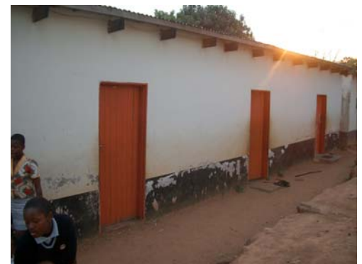
Top: There is a variety of different standards of construction in the informal settlements around Mbabane.
