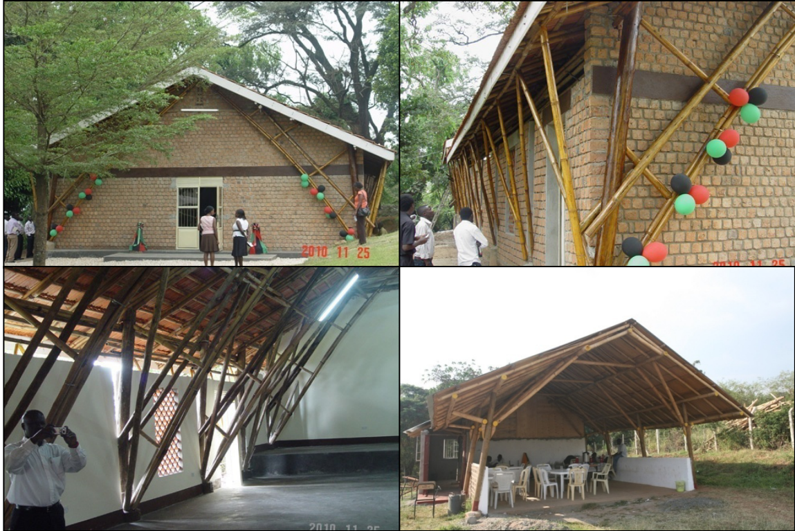
Picture 4: Finished bamboo structures in Uganda (top row and bottom left) and Kenya (bottom right)
