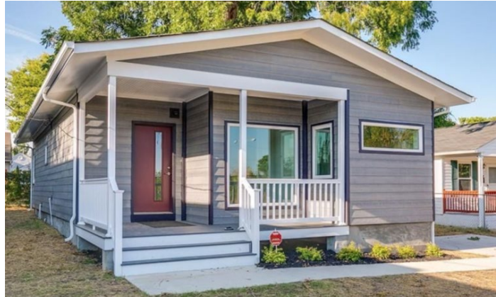
Figure 32: Completed indieDwell Home
