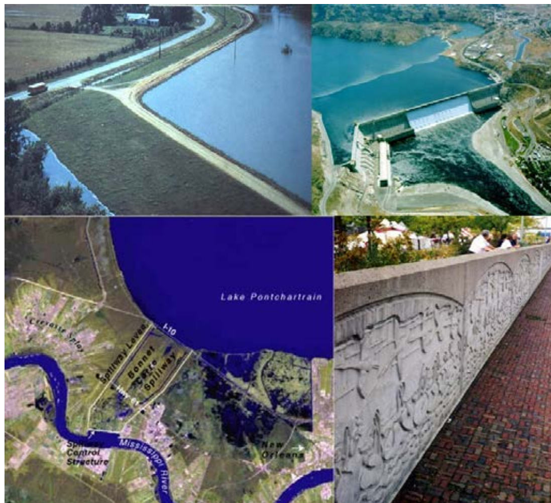
FIGURE 2.4 Structural Flood Mitigation Measures, clockwise from top left: Mississippi River levee; Grand Coulee Dam on the Columbia River in Washington; a floodwall in which protects the city Winona, Minnesota along the Mississippi River; and the Bonnet Carré Spillway, a floodway that diverts water from the Mississippi River into Lake Pontchartrain to reduce the flow passing New Orleans.
