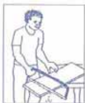
Saw and nail boards to make strong shutters
