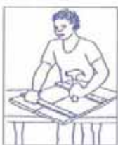
Saw and nail boards to make strong shutters
