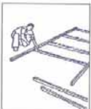
Nail studs to top and bottom plates on the ground
