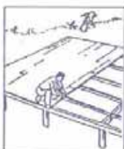
Nail floor boards to joists
