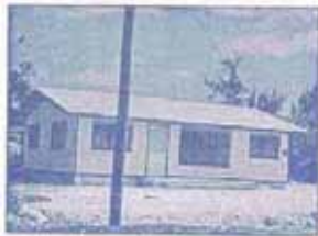
Wood frame house in Nuku'alofa, Tonga
