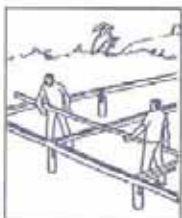
Put floor joists in place
