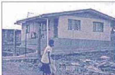
Concrete Block house in Suva, Fiji
