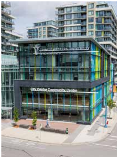
Accessible Route Highlighted by Paving Contrast.
