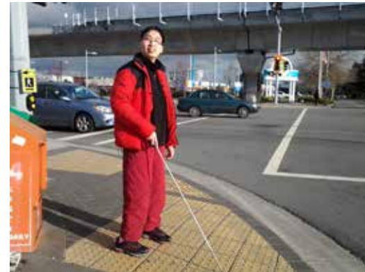
Barrier-free design incorporates a clear accessible path with cane detectability and good colour contrast.
