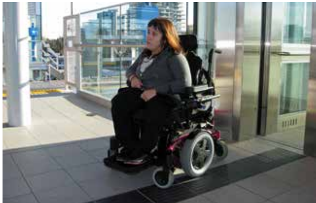
Accessibility is enhanced at elevators by providing a contrasting floor colour to delineate the accessible path. Similar flooring contrasts should be considered to delineate the path to entrances, or other strategically important pathways.
