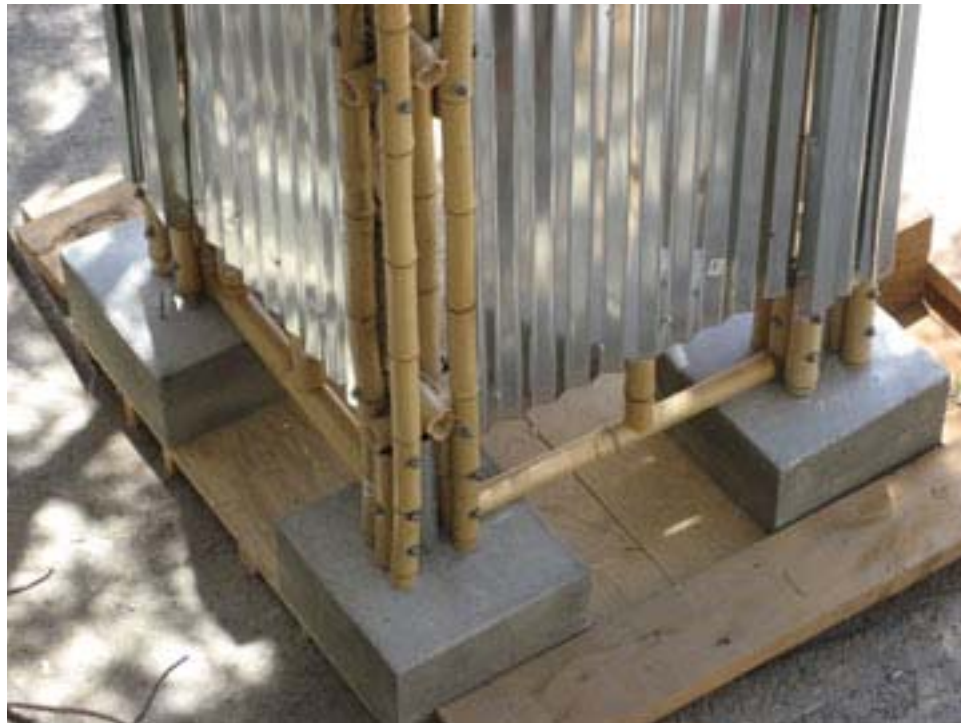
Figure 5.15 Lower external portion of the prototype showing three precast concrete footings and uncovered parts of the column system. Source: Photograph by Author.
