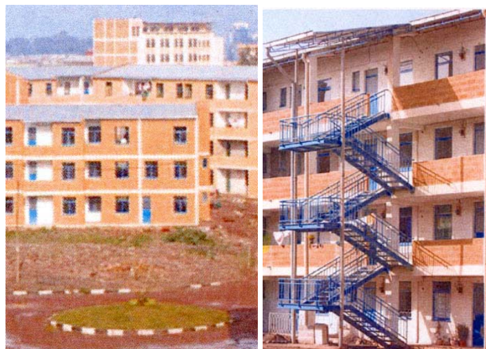
Figure 2.2 The Condominium Housing Project: project co-developed and built by Ethiopia's Housing Development Office (HDO) and the German Technical Co-operation (GTZ). Source: Low Cost Housing: Technical Manual by German Technical Co-operation.
