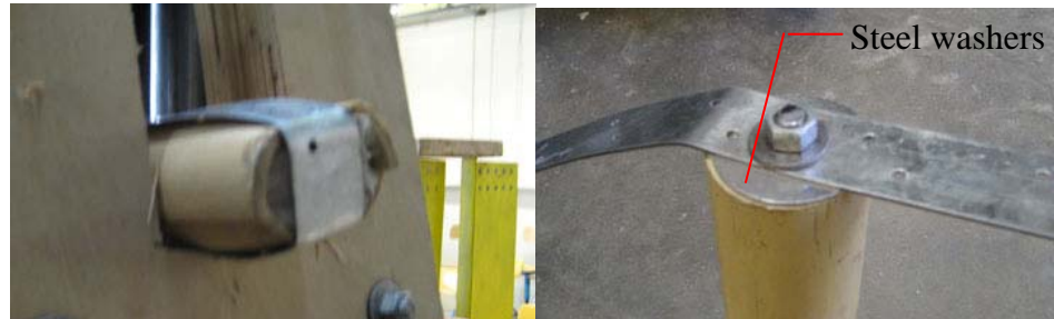
Figure 6.3 Left: Steel strap reinforcement crushing the end of bamboo pole. Right: Steel washer used to prevent steel strap crushing the end of bamboo pole. Source: Photograph by Author.
