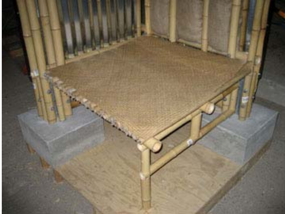
Figure 5.14 Lower portion of the prototype showing a floor system and decking constructed from 1 inch poles and woven mat covering. Source: Photograph by Author.
