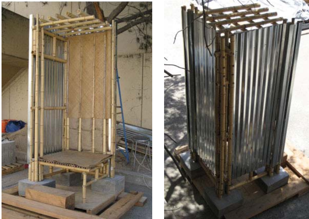
Figure 4.4 Prototype: a full-scale section of the proposed low cost housing unit. Source: Photograph by Author.
