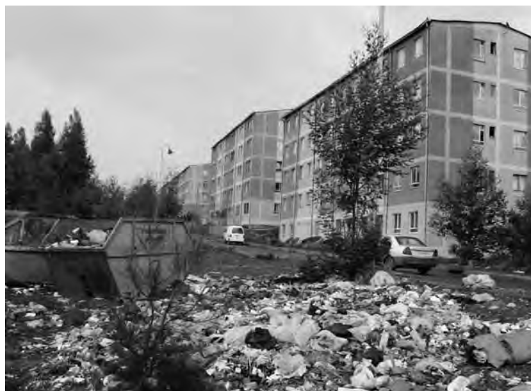
Figure 30: Accumulated rubbish adjacent to condominium buildings Mikililand condominium site, Addis Ababa.
