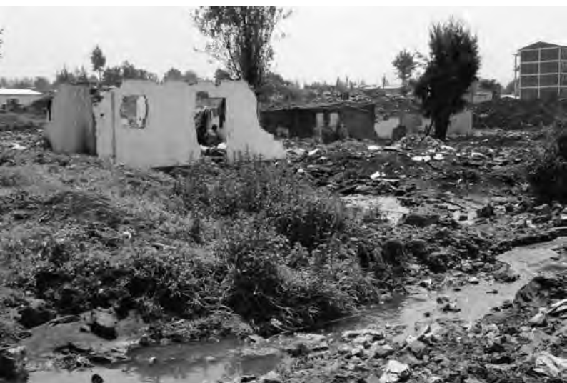
Figure 25: Lideta site being cleared. © UN-HABITAT/ Katherine Hegab
