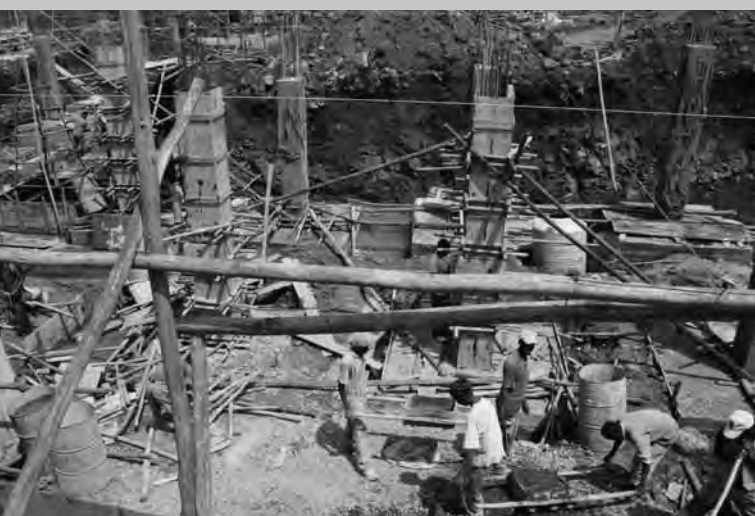
Figure 11: Multi-storey buildings in Addis Ababa are typically constructed from cast in-situ reinforced concrete frame with brick infill walls. © UN-HABITAT
