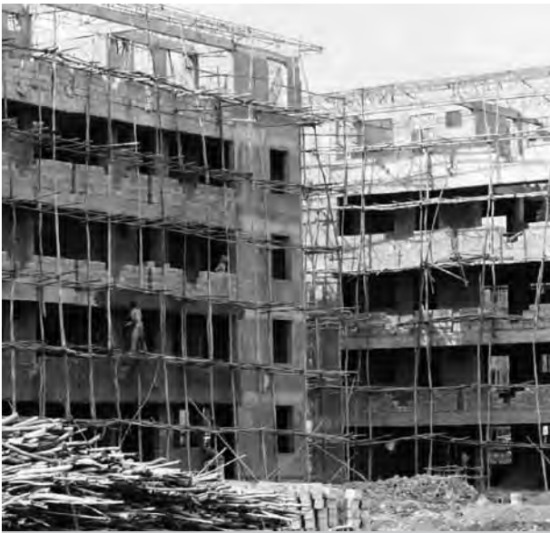
Figure 18: Bole Summit under construction Addis Ababa. © UN-HABITAT/ Katherine Hegab
