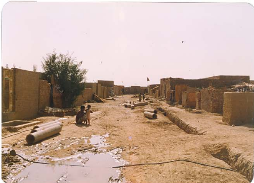
Laying of services.
