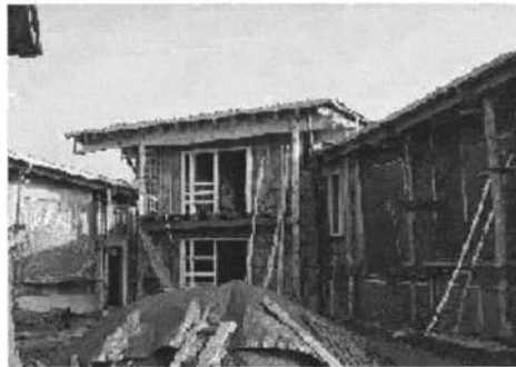
Figure 7 SB building in Warns (picture during construction in 2003 October)
