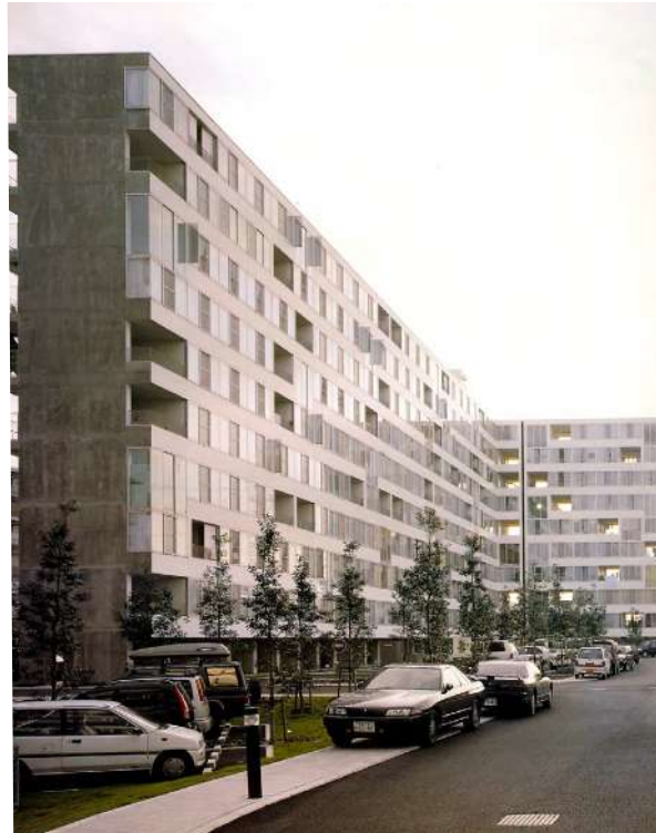
Gifu Kitagata Apartment Building; Gifu Prefecture.
