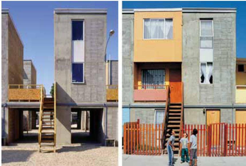
Figure 2: 36 m 2 initial + 36 m 2 self built units in Quinta Monroy, Chile.
