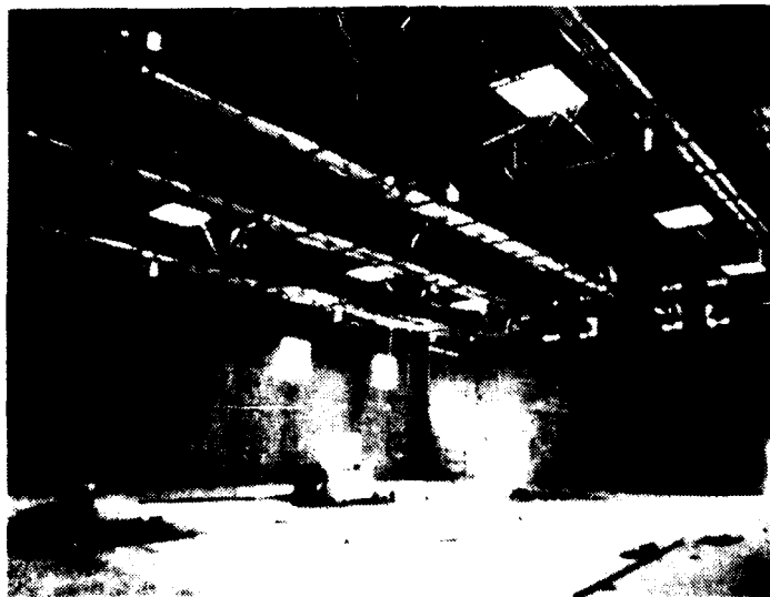
Figure 4. Interior construction—Fort Bliss.
