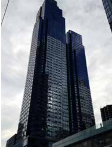
Figure 11. 75 West End Avenue
