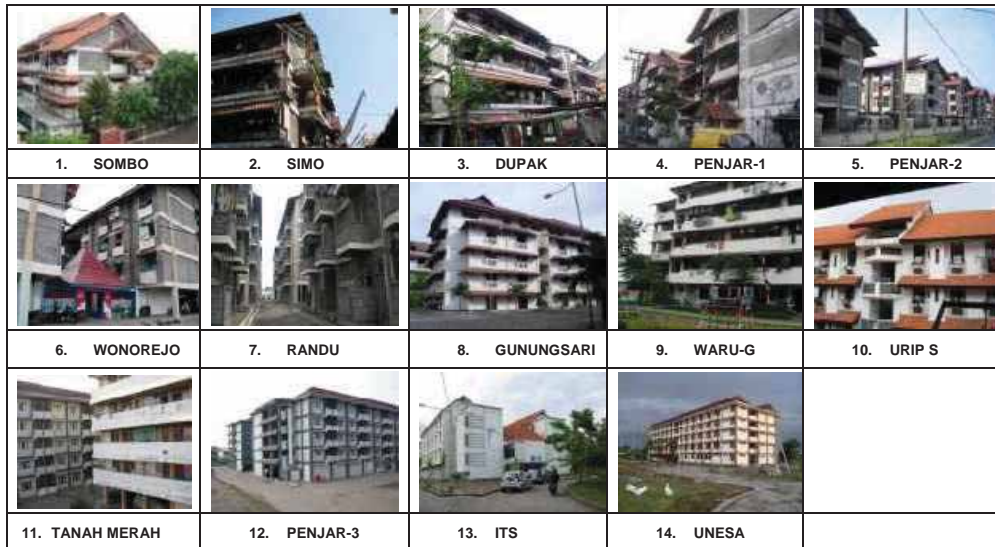
Figure 3- 1: Performances of the building population, in which the units and low income households are taken as samples
