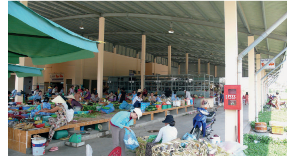
Sheltering informal economies — The large roof of the hawkers’ market simply and cost-effectively accommodates local trade activity.
