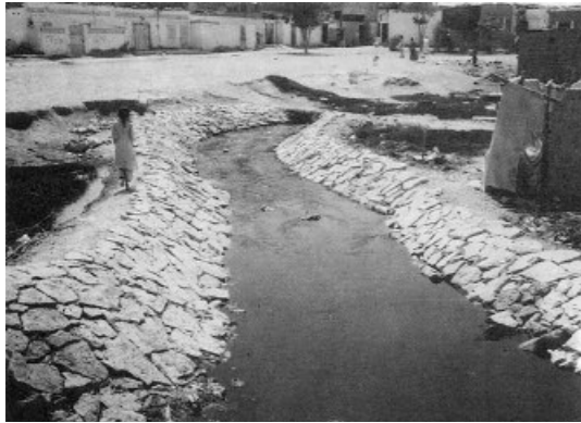
The use and abuse of nallahs — Ad hoc sewage lines leading to nallahs , the nearest natural drains, were gradually replaced with a proper underground system. Silting, proneness to flood and general pollution have threatened the nallahs and induced the realization of trunk sewers and treatment plants. Today, covered nallahs are a common feature of Karachi's urbscape.
