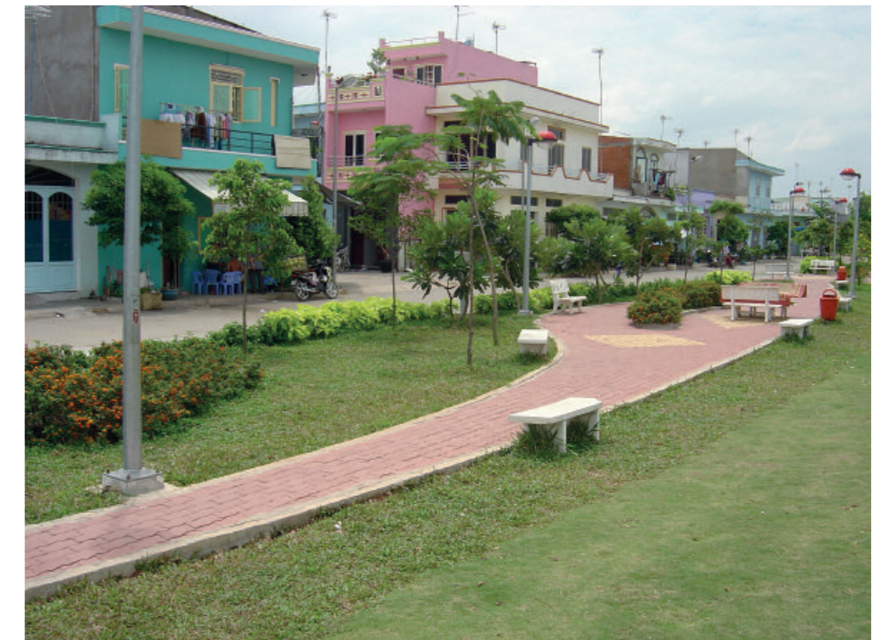
Aerated lagoon linear park — The edge of the aerated lagoon was designed as a community park for the sites-and-services housing relocation area.
