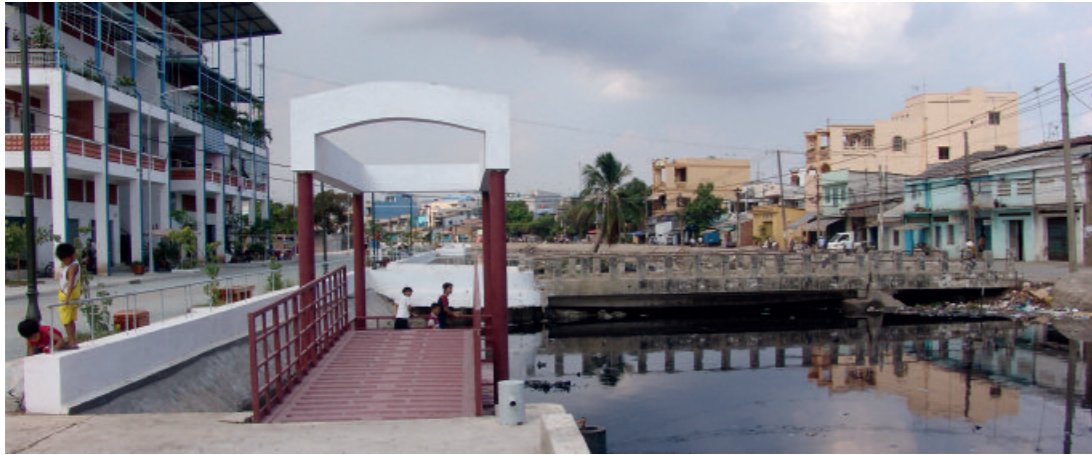
Reconfigured canal edge — The widened and newly embanked canal was equipped with a boat launch.
