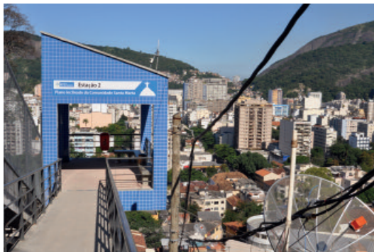
Navigating difficult terrain — The program invested substantially in pedestrian infrastructure provision.
