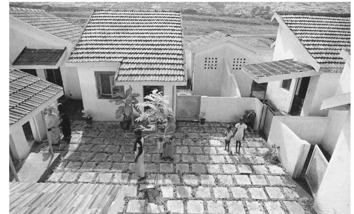
Clusters and courtyards — Despite the project’s relatively small site, every home was provided with both its own private “open-to-sky” space and a shared courtyard.
