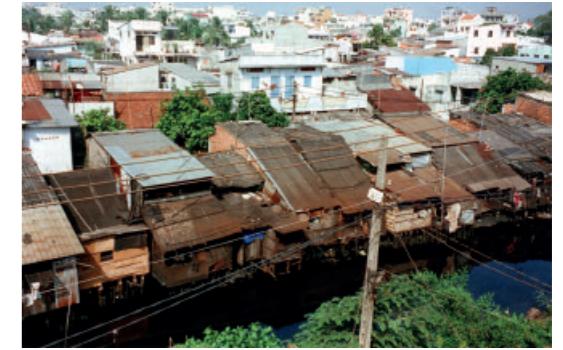
Encroached canal — New rural residents to the mega-city tend to settle along canals and other low-land areas.
