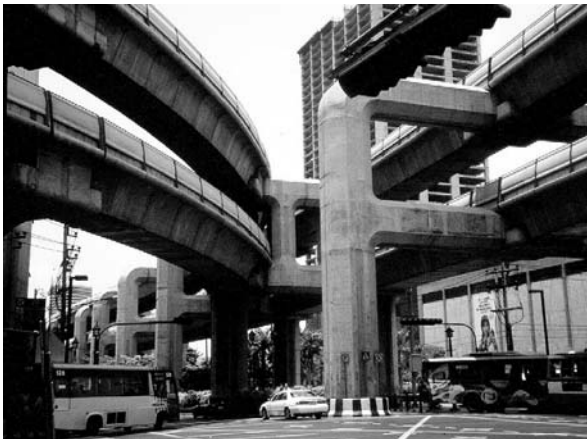
Fig. 3. The massive structure of the Skytrain's line and stations over Bangkok's streets (Source: Mike Jenks)
