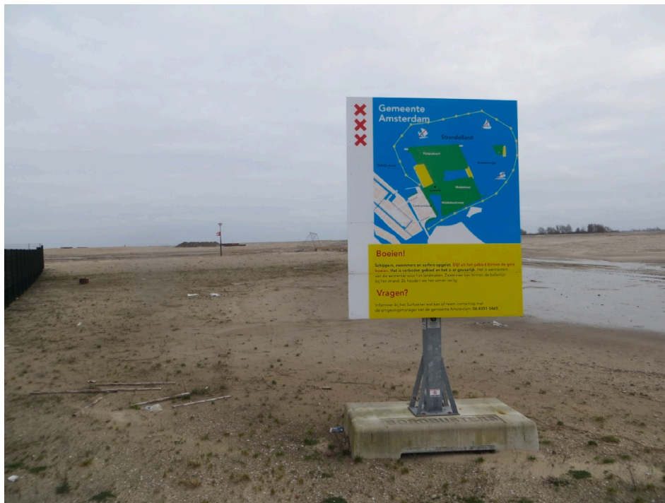
Fig. 2. Land preparation in Strandeiland, Amsterdam. Around 8.000 new homes will be built before 2040 and in accordance with the negotiated scheme of '40-25-35.' Source: Photo taken by Bob Wijburg.
