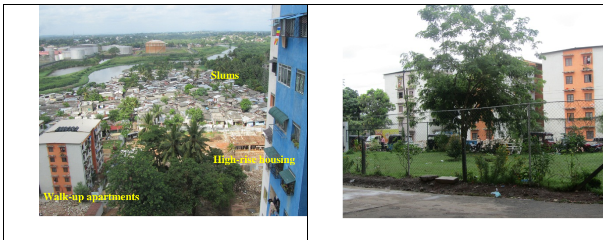
Figure 7.4 : Walk-up apartments adjoining Sahaspura and slum area
