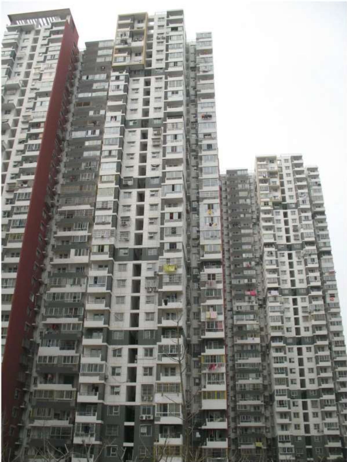
Figure 5. Low- cum -medium price housing project at Lianhuacun, Nanjing. Source: Author, March 2015.
