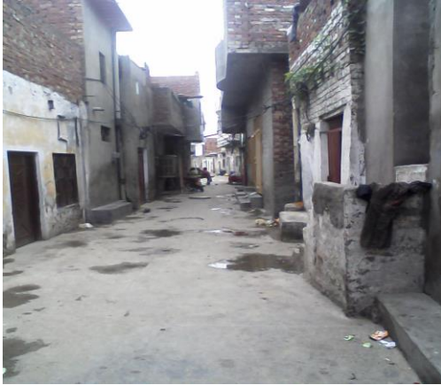
Fig 4.7: cement paved street in tanki no. 56
