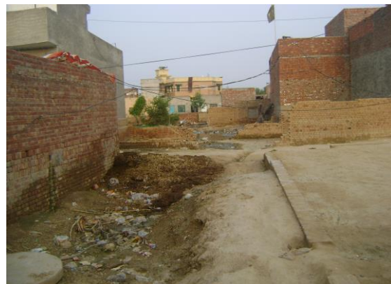
Fig 4.5: House structure in badar colony
