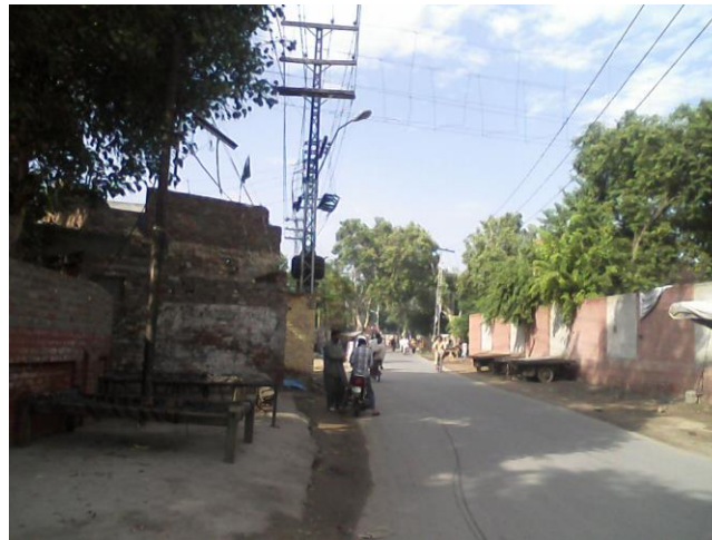
Fig 4.9: Street lights in Tanki no.56
