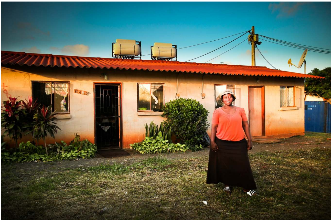
A resident stands in front of her home which has undergone a 'green upgrade'. The solar water heaters for two homes are seen on the roof behind her.
