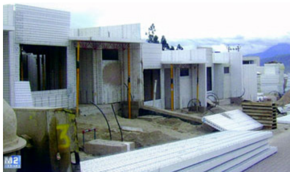
Figure 2. Panel building system installation
