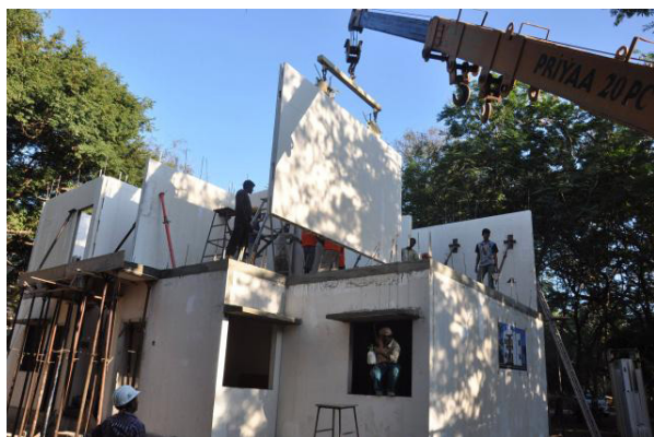
Figure 1. GFRG panel installation.
