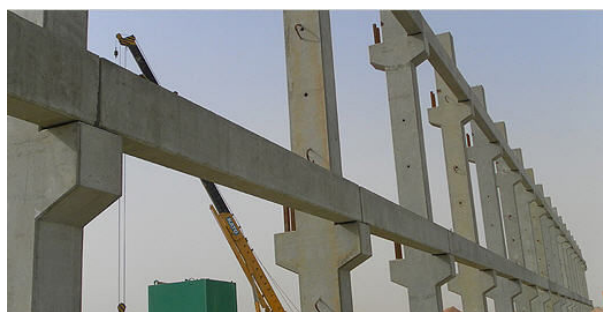
Figure 3. Precast, pre-stressed and prefab installation.
